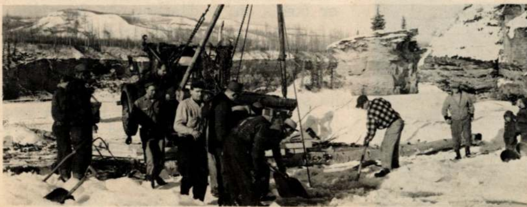
RAISING POLLON & GOODVIN CRAWLER WHICH PLUNGED THROUGH ICE ON PEACE WHILE CLEARING RIVER OF SNOW FOR CROSSING OF B. OF T. MOTORCADE DRIVE FOR HUDSON'S HOPE-CHETWYND HIGHWAY IN 1958. PETE GOODVIN IN CHECK JACKET WENT DOWN WITH MACHINE, WAS SAVED BY BUD STUART, LEE PARSONS AND PETE MACDOUGALL
